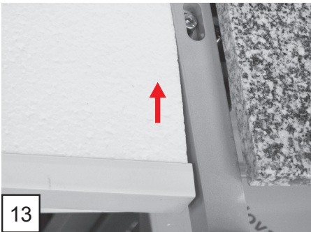
13 Putting insulation under working top
