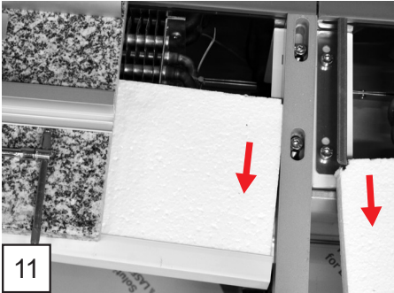
11 Removal of insulation under the working top
