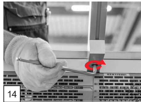
14 Screwing lamp rack
