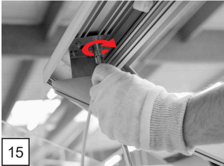
Screwing lamp profiles
